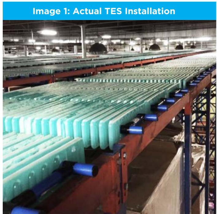
As ambient temperatures increase during peak hours of the day and the heat rejection of the condenser is less efficient, the control algorithms reduce or stage the run time of the refrigeration system and allow the fully charged TES modules (frozen PCM) to absorb the heat infiltration and maintain temperature stability inside the freezer.
